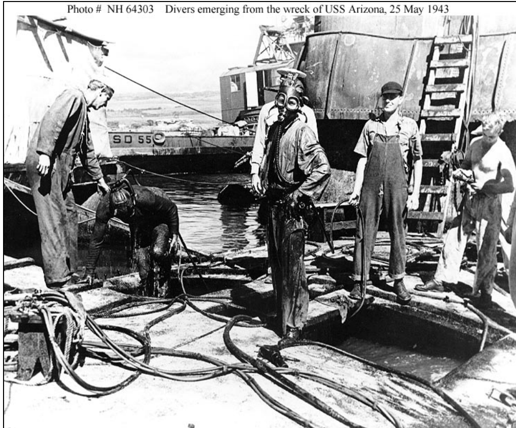
Figure 3.11. Diver on Arizona deck, 1943. Note shallow water diving equipment made from gas mask (USS Arizona Memorial Archive Photo).
